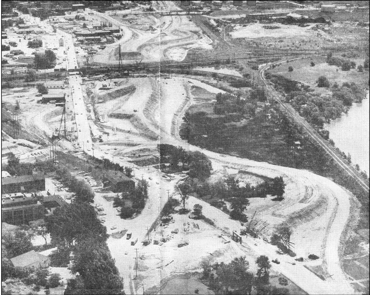
Figure 2.4.6-13. 1958 Aerial Photograph during Construction of the Oswego Boulevard Expressway. Linking the Oswego Boulevard Expressway with Interstate 81 north of the city required significant earth disturbance and construction of earthen berms to navigate the landscape and poor soils closer to Onondaga Lake (Hoffman, 1958b; collections of the Onondaga Historical Association)
