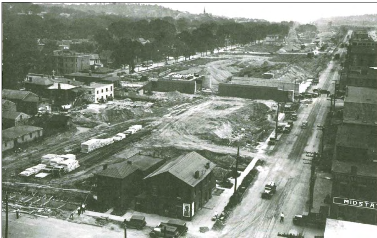
Figure 2.4.6-3. ca. 1935 View of Construction of Elevated Railroad Right-of-Way. This ca. mid-1930s view from McBride Avenue looking east depicts the construction of the elevated New York Central Railroad right-of-way between Burnet Avenue (depicted as a tree-lined street on the left of the frame) and Canal Street (on the right of the frame). Note the considerable ground disturbance as well as the houses that were later removed for construction of the railroad right-of-way, which was common within all parts of the elevated right-of-way that would later become Interstate 690 in the 1960s. (CNYCNRHS, 1986)
